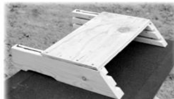
Figure 3. TOP FRONT is assembled and beveled edges are flush, matching the sloped roof.
